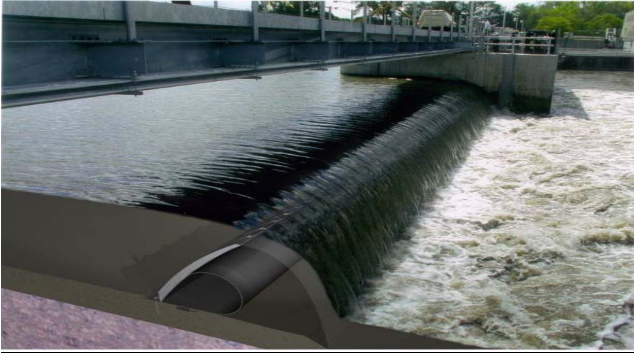
Slide -12 Obermeyer Flashboards
